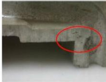
Casting defect
